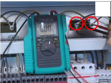
7. Measure ~volts on all heaters (700 series = 10 heaters and 800, 900 = 14 heaters) there should be no voltage
