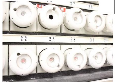
3. If you have external circuit fuses. Check and replace broken fuses
