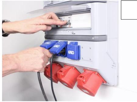
2. Turn OFF breakers/fuses or unplug the oven before opening the ovens electrical panel
