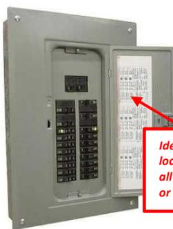
1. In your **electrical circuit box**, check and identify the position of all the external circuit breakers or fuses for the oven
